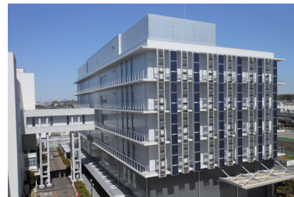
Solar panels on the wall of a building of Nikon Yokohama Plant
