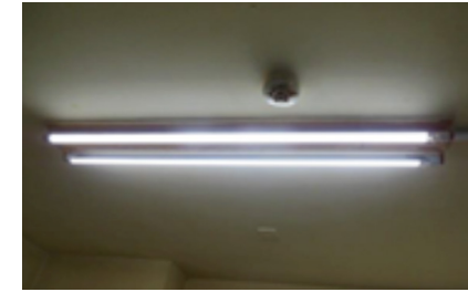
Fluorescent-style LED lighting in common areas at Nikon Imaging (China) Co., Ltd
