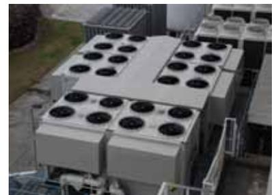
Heat pump chiller equipment of the seamless HVAC system (Tochigi Nikon Precision)
