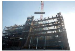
Ceremony of putting up the ridge beam (September 2023)
