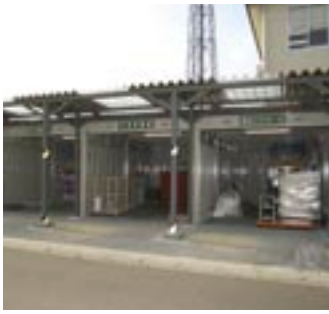
Sorting and reduction of waste volume has been achieved at the Sendai Nikon Recycling Center through the use of special machines.
