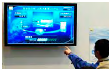
Monitor showing the amount of power generated in real time at Nikon Kumagaya Plant
