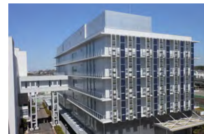
Solar power generating equipment on the wall of a building of Nikon Yokohama Plant
